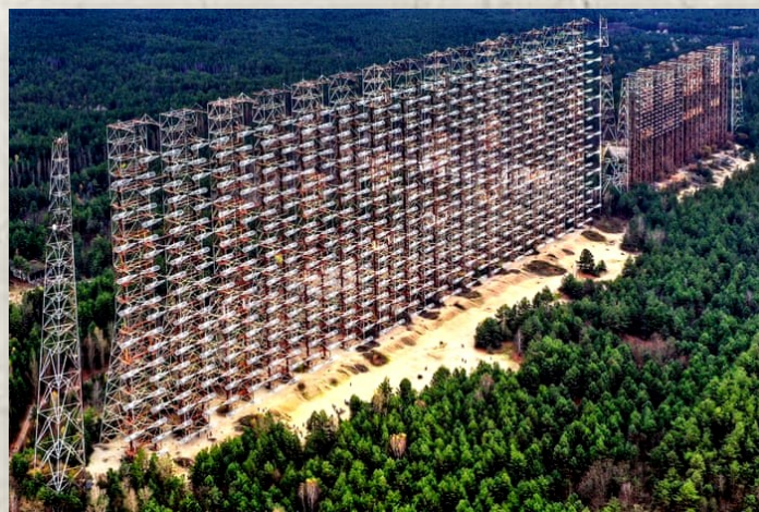
The massive Chernobyl Duga antenna array—2300 feet long, 700 feet tall—in its time, it was one of the largest antenna arrays ever built on earth Photo: Wiki Commons
