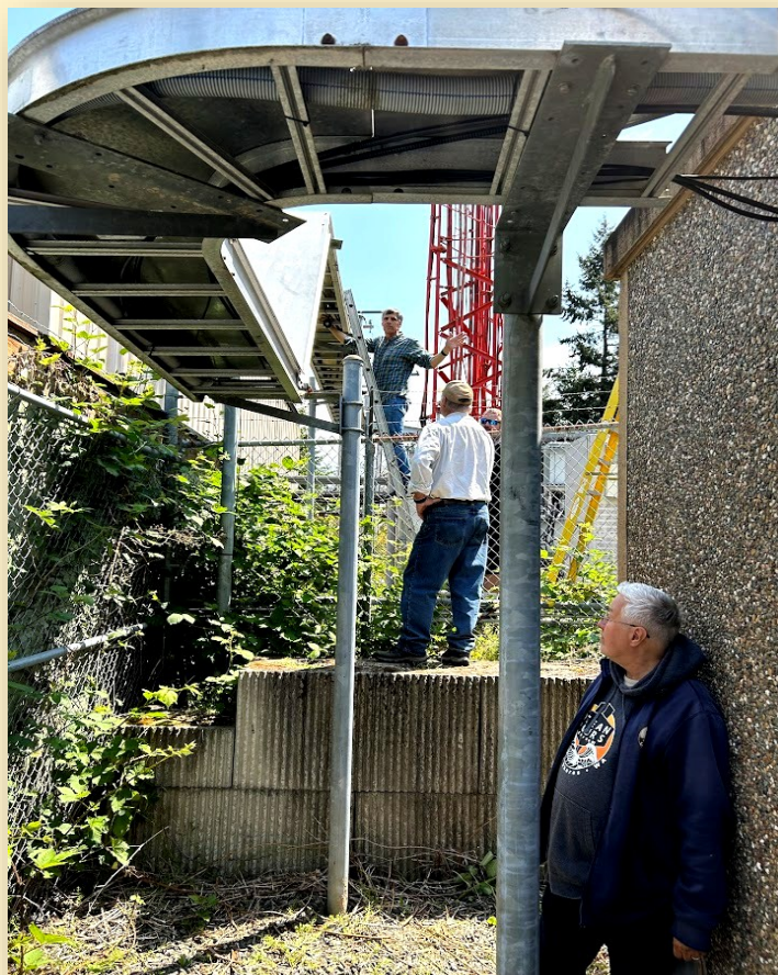
The Radio Club of Tacoma Repeater Committee at the base of the Bates repeater shared tower—one of the tallest broadcast antennas in Tacoma, at 692 feet with the W7DK antenna at about the 600 foot level. L>R: Dan KD7SV , Mike W7MKE (back to us) and Nick K7MO (SK March '25)
