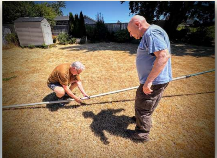
Once on the ground, it was easy enough to re-attach the fiberglass tubing sections and cinch them down again, ready to re-erect the vertical
